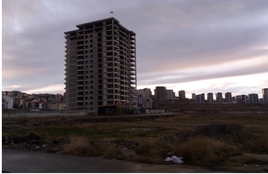
Figure 12: New multistory apartment buildings in Yükseltepe Source: Taken by the author, 2019
